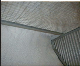
Unit walls are custom-molded to the cave wall.
